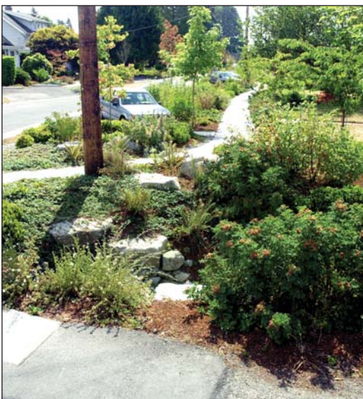
Rain gardens and natural swales being used instead of storm drains and pipes.
