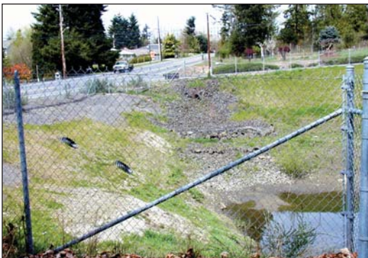
Traditional storm water pond.
