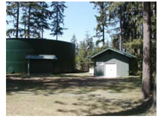
City of Langley water reservoir
