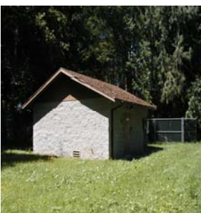
City of Langley water pump house
