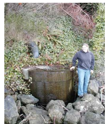
Park Avenue storm interceptor
